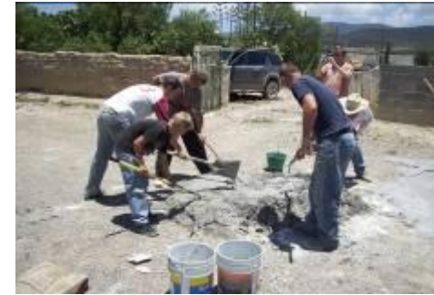
Nathan Weaver, Marc, Jordan and Logan Sankey, Steve and Kent Stetler mixing concrete by hand for church repairs in La Boca.
